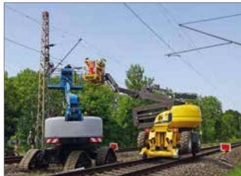
Construction of contact lines
