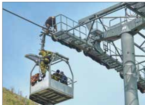
Cable car construction
